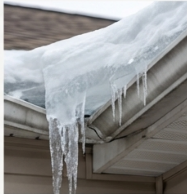
Sagging gutters filled with ice
