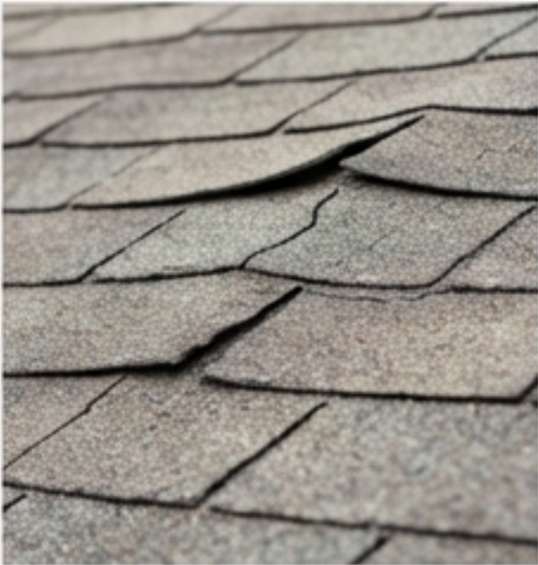
Curling or cracked shingles
