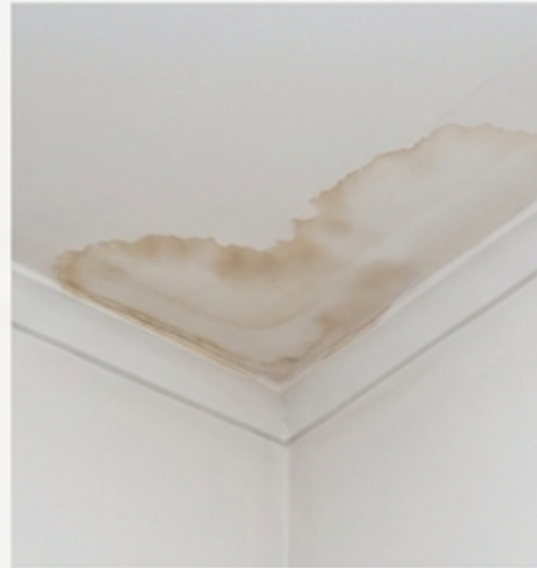
Water staining on ceilings
