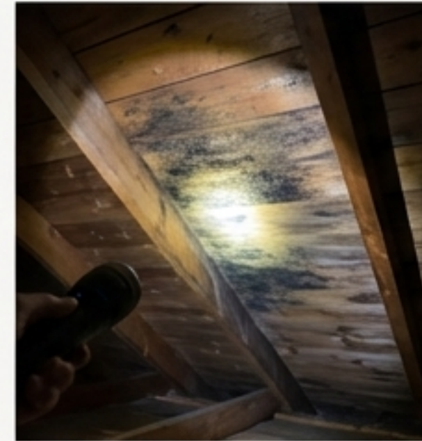
Mold or mildew in attic spaces
