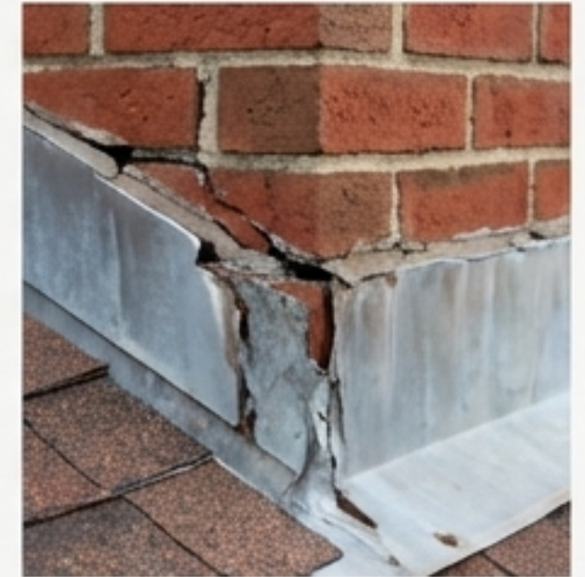
Loose or degraded flashing around chimneys and vents
